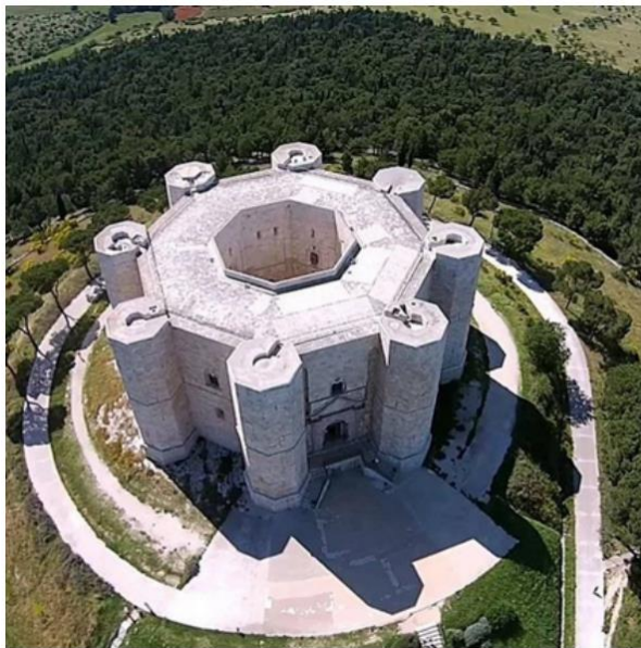
(a) Aerial view
